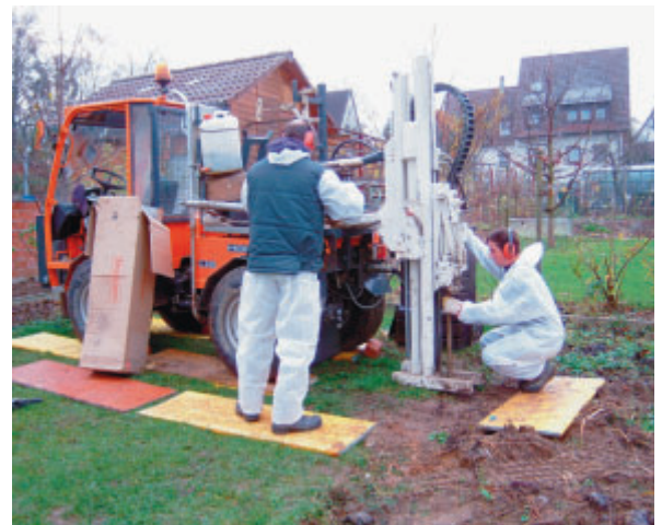
In-situ remediation with nanoscale iron particles
