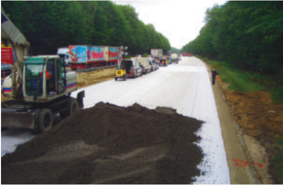
Prepared substructure for a concrete road surface
